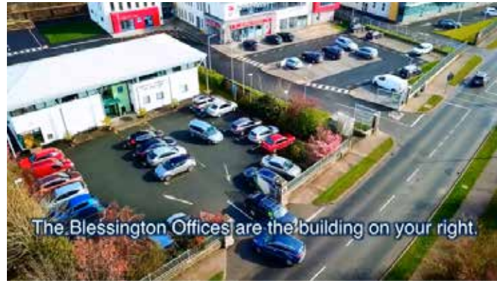
Aerial view of the Blessington Offices
